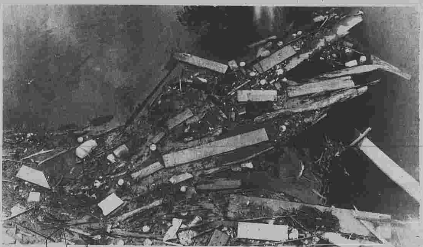
DEBRIS AT UNION POND DAM.
