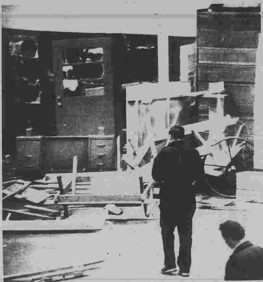
State Police Crime Squad investigators Wednesday, after six guards were injured examining debris in the gym of the Connecticut maximum-security prison in Somers during a disturbance at the facility.
